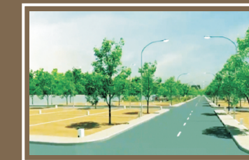
Road, Water Drain & Pathway
